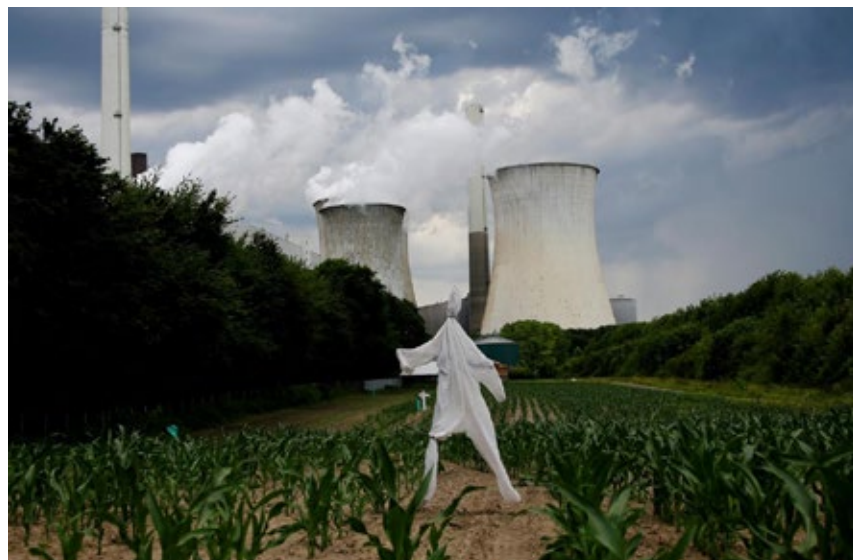
A scarecrow stands in a corn field in front of the Neurath coal power plant of German utility RWE in Neurath, west of Cologne
