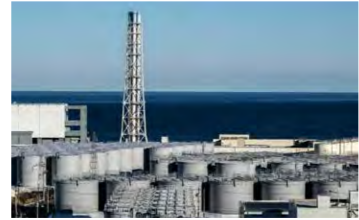
A general view shows storage tanks for contaminated water at the Tokyo Electric Power Company's (TEPCO) Fukushima Daiichi nuclear power plant
