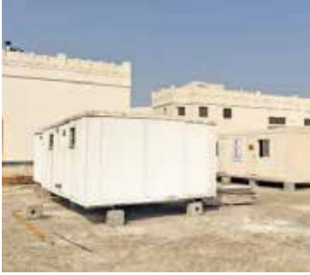
Three permanent maintenance cabins installed at the Al Ramli housing area after the August 18 fire
