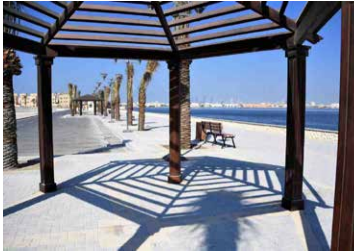
A walkway project
