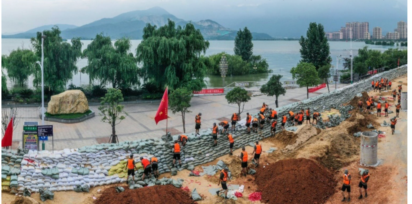
Chinese soldiers erect a sandbag barrier along the shore of Poyang lake after heavy seasonal rains in Jiujiang, in China's central Jiangxi province
