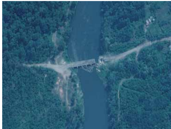
A satellite image shows a close up view of a damaged bridge, in Rubizhne, Ukraine
