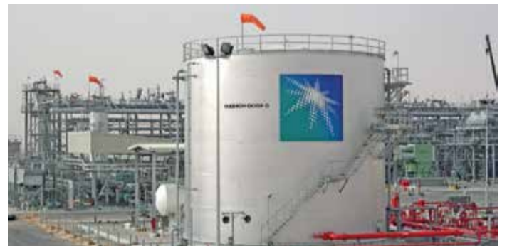
A general view of oil tanks at a plant in Haradh, about 280 kilometres (170 miles) southwest of the eastern Saudi oil city of Dhahra
