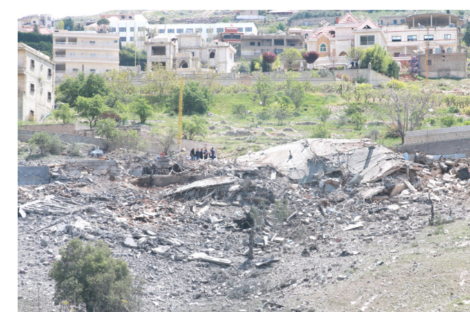
A general view shows a destroyed building targeted by Israeli air strikes on the village of Nabi Sheet in the Baalbek district in Lebanon's eastern Bekaa Valley
