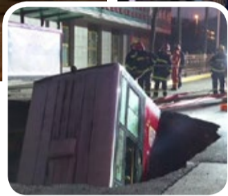
The sinkhole opened up at a bus stop in Xining, north west China
