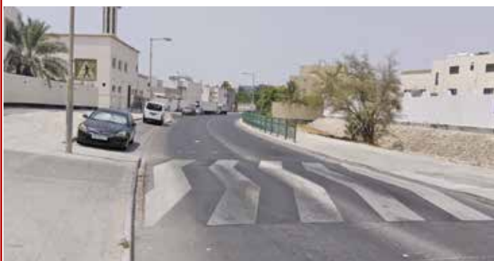
Speed bump on Road 5 in Hamad Town's Block 1205
