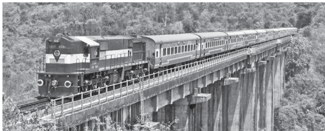
Konkan Railway is undoubtedly an engineering marvel.
