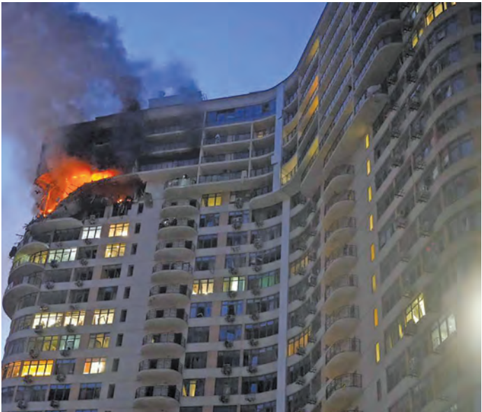
Multi-storey residential building with an ongoing fire at damaged high levels following a strike in the Ukrainian city of Odesa, amid the Russian invasion in Ukraine.
