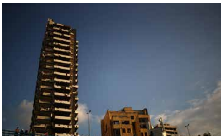
A view shows damaged buildings near the site of the blast at the Beirut's port area, Lebanon
