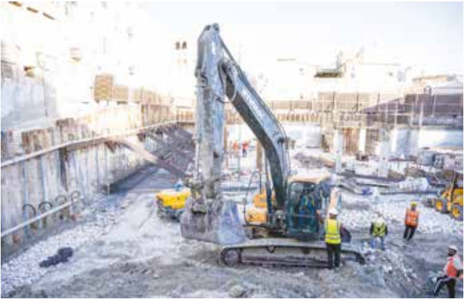
A construction site of Muharraq Development Phase One
