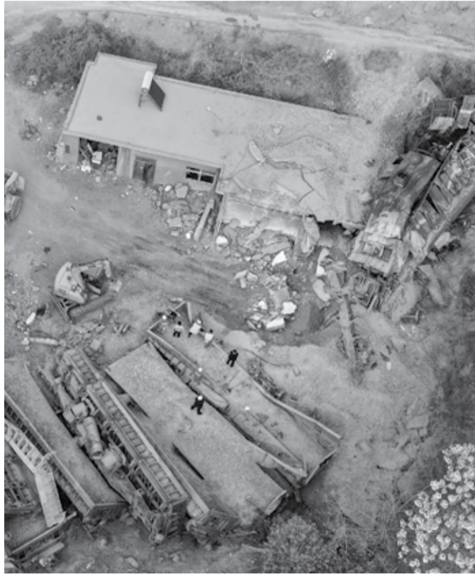
Rescuers searching at the site where a train carrying aluminum ore derailed and hit a village house in Zhengzhou in China's central Henan province.
