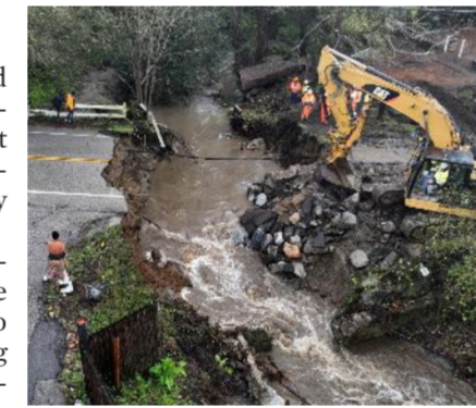
Workers make emergency repairs to a road that was washed out
