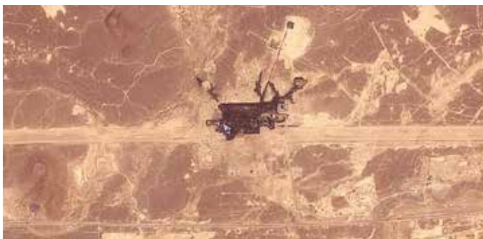
Satellite image taken by Planet Labs PBC on September 11, 2026 shows a general view of an infrastructure site southeast of Medina along the general route of Saudi Arabia's East-West pipeline (Petroline) after it was damaged by fire
