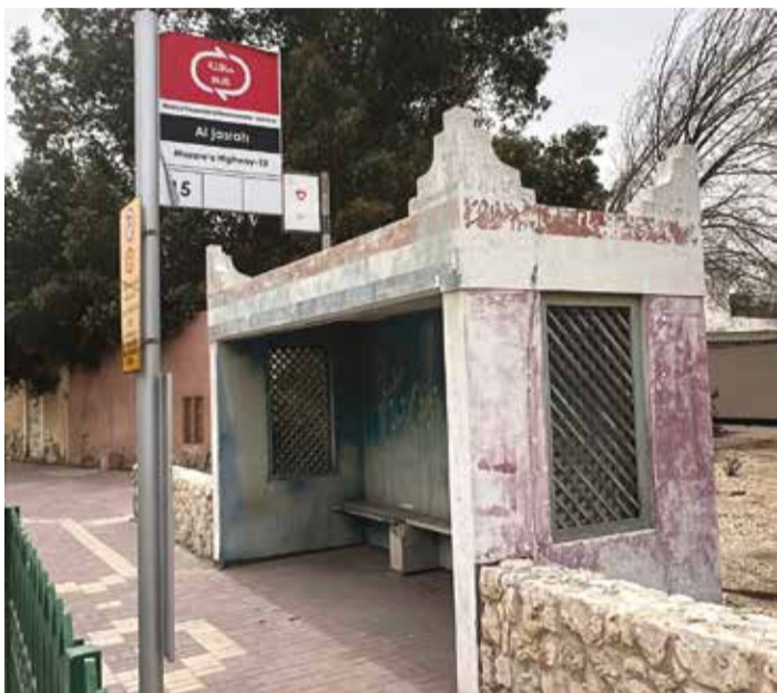
A bus stop that needs an upgrade for public convenience
