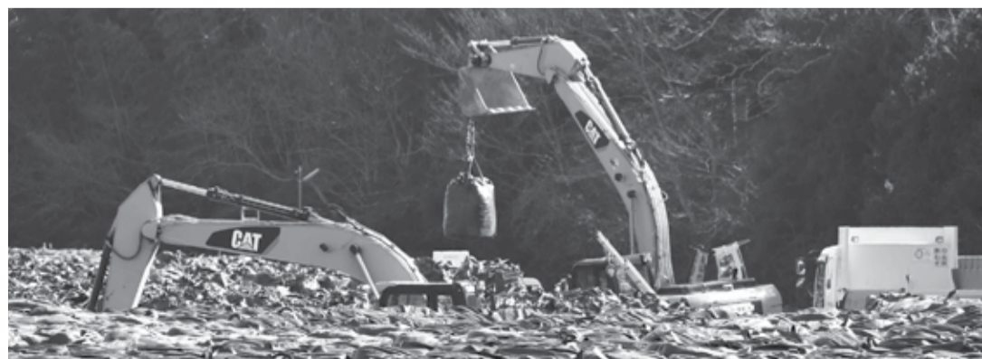
Excavators piling nuclear contamination at a temporary place in Tomioka, Fukushima prefecture.
