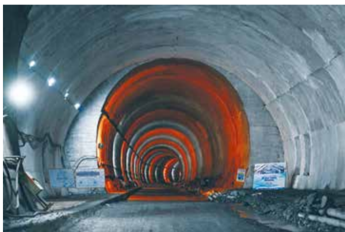
The Zojila tunnel, India's longest road tunnel project connecting Jammu and Kashmir state with the Ladakh region
