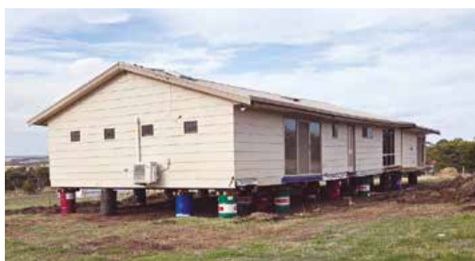
A house getting ready to be moved to its correct location after being built on a neighbouring section, in Camperdown, west of Melbourne
