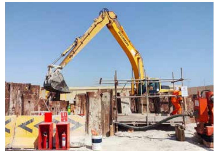
Excavation work in the area
