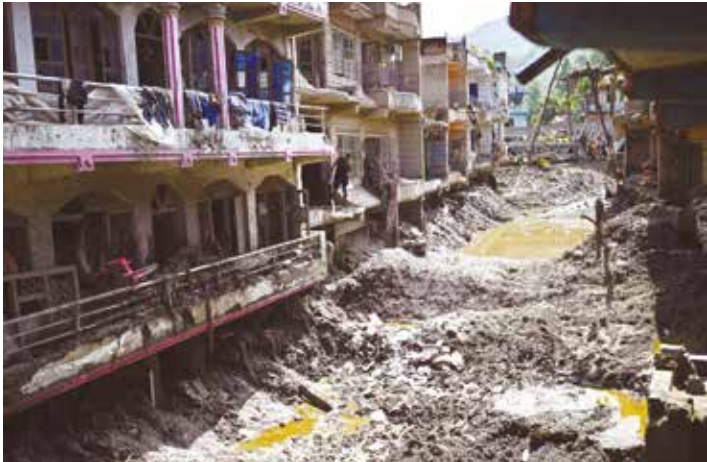
A man looks at the remains of sludge-ridden houses in the aftermath of flash floods at Devighat in Nepal's Nuwakot district
