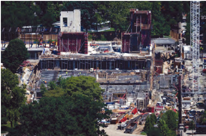
A view of the ongoing construction of a planned ballroom at the White House, as seen from the Washington Monument observation deck in Washington, DC
