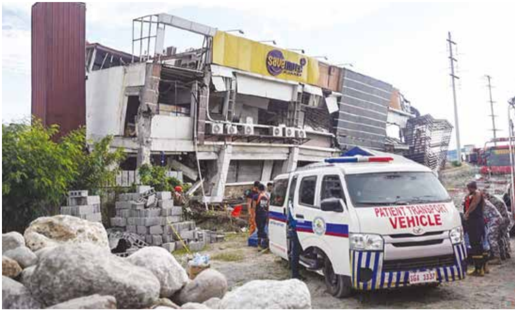
Responders conduct a rescue operation at a collapsed building after a 7.8 magnitude earthquake in General Santos City
