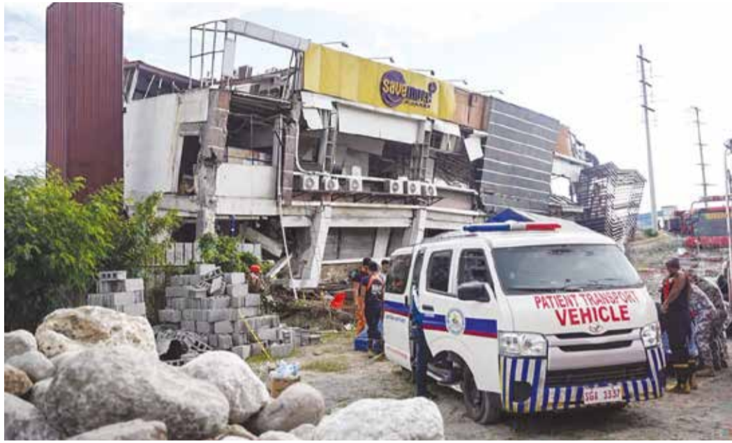
Responders conduct a rescue operation at a collapsed building after a 7.8 magnitude earthquake in General Santos City
