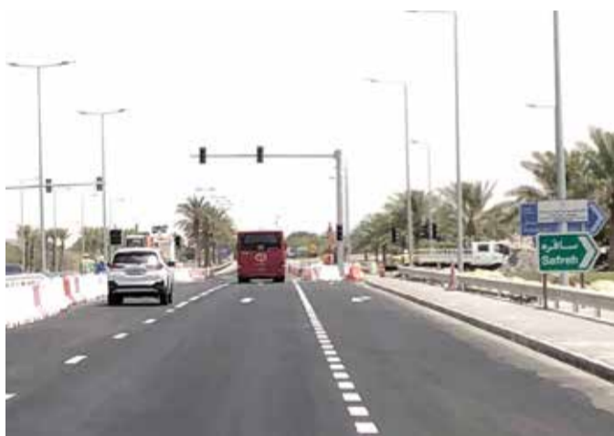
The General Traffic Department at the Ministry of Interior announced the commencement of operations for a new traffic signal today at the intersection of Sheikh Salman Street and Road 4225 in the Safra area of the Southern Governorate. To ensure the safety of everyone, the directorate advises citizens and residents to strictly adhere to the traffic rules.
