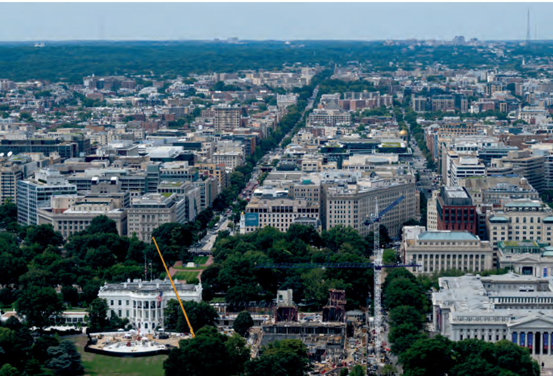
Construction of the new helipad on the south lawn and the ballroom that will replace the East Wing of the White House, is seen from the observation deck of the Washington Monument in Washington
