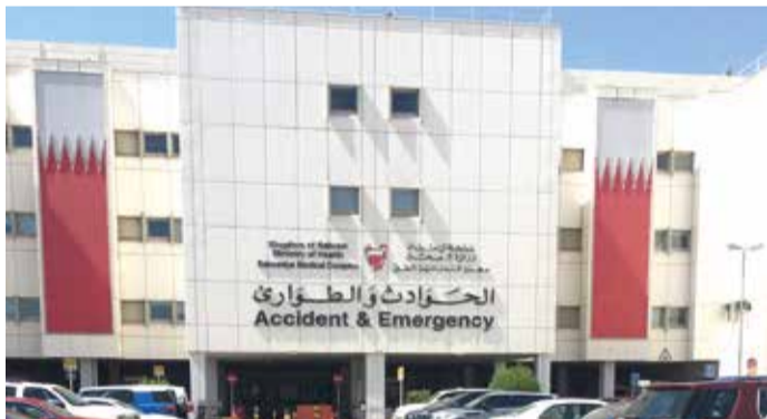
Ongoing project aims to improve infrastructure, facilities and services at the hospital
