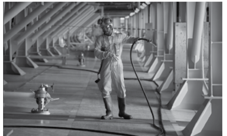
A worker works with a hose on the Kaombo Norte, an oil tanker converted into a FPSO vessel (Floating Production Storage and Offloading),
