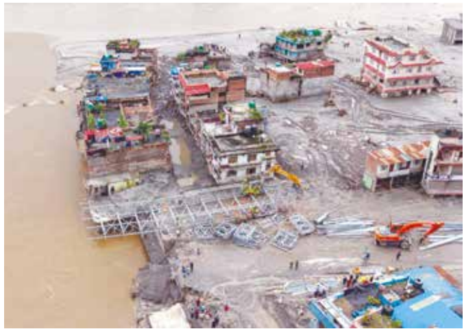
An aerial view shows Army personnel building a bridge over the Tadi River in the aftermath of flash floods in Devighat, Nepal’s Nuwakot district
