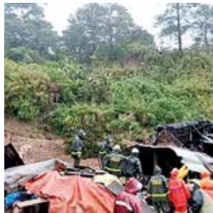
Rescuers working at a landslide site
