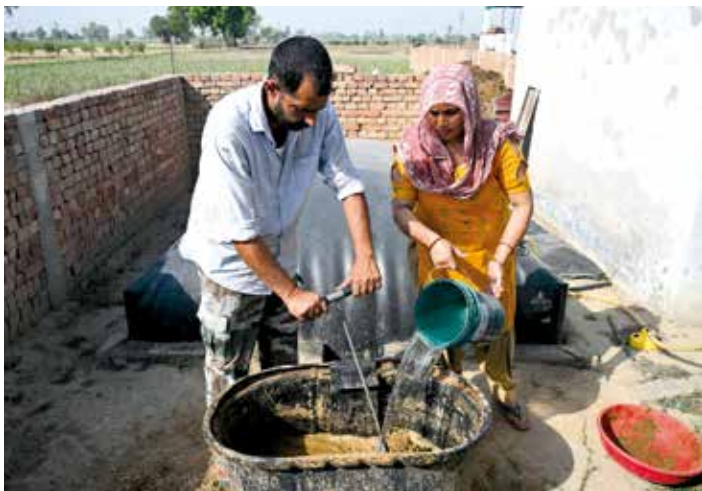
Residents pour cow dung into their biogas plant at a village in Uttar Pradesh
