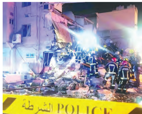
The Arad building collapsed after a gas explosion on February 12, 2025
