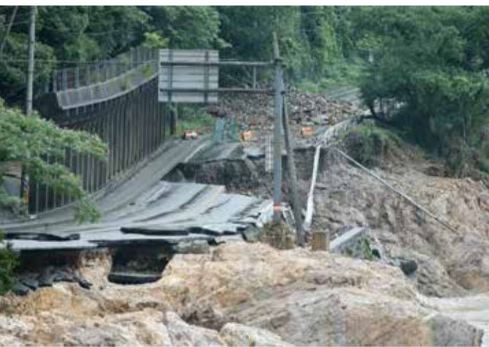
The torrential rain destroyed roads and bridges, cutting off isolated rural communities
