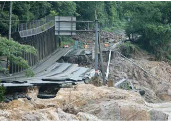
The torrential rain destroyed roads and bridges, cutting off isolated rural communities
