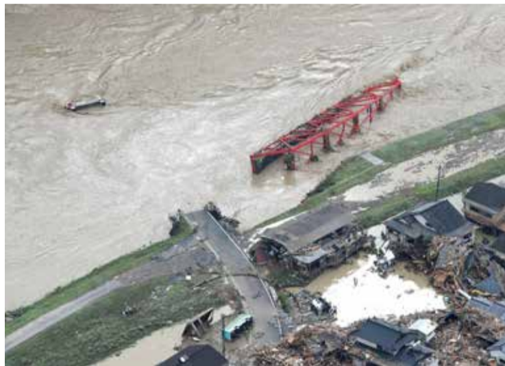
The floods washed away bridges
