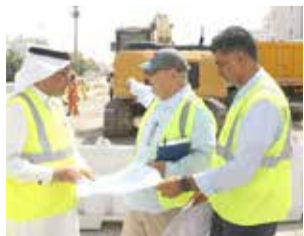
Al Farea inspects the sanitary drainage project
