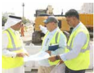
Al Farea inspects the sanitary drainage project
