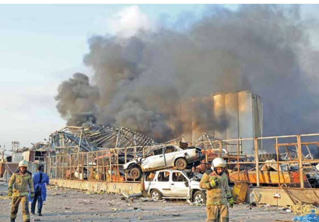
Above and right, views of the damage caused by the blast
