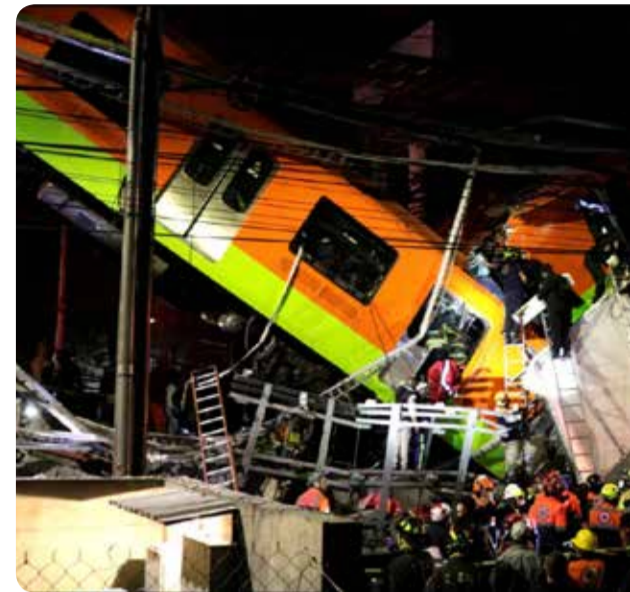
In pictures, rescuers work at a site where an overpass for a metro partia
