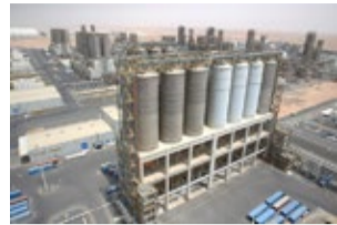
General view of the Borouge petrochemical facility at ADNOC's Ruwais Industrial Complex in Ruwais, United Arab Emirates
