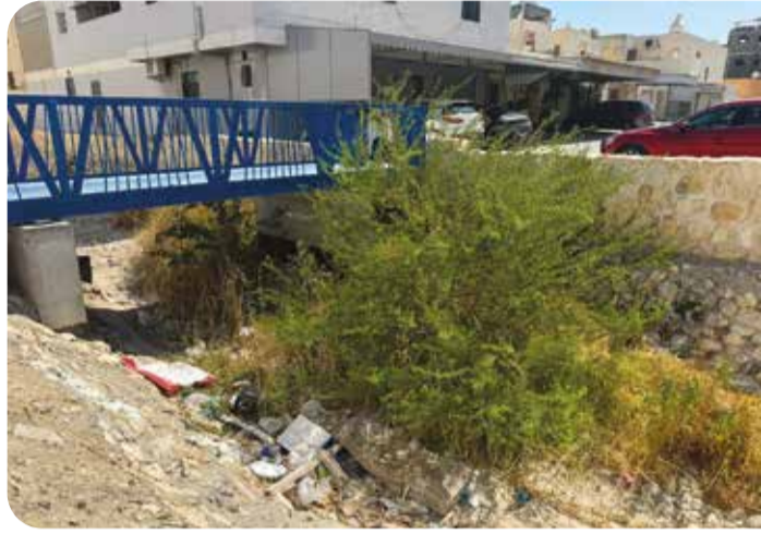
Blocked drainage channels clogged with vegetation and dumped waste are seen during a field inspection in Hamad Town.
