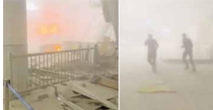
Extensive damage at Kuwait International Airport's T1 building following Iran's missile and drone strike overnight.
