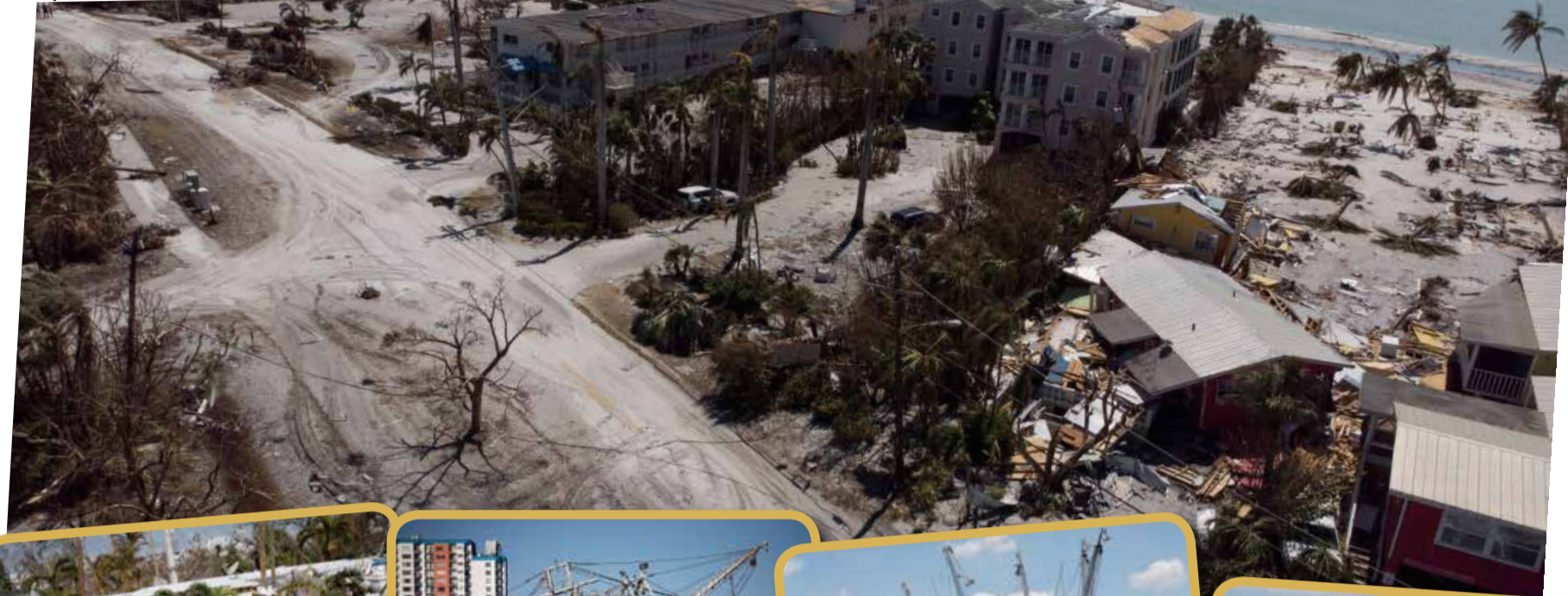
Destroyed buildings are seen after Hurricane Ian caused widespread destruction in Sanibel Island, Florida
