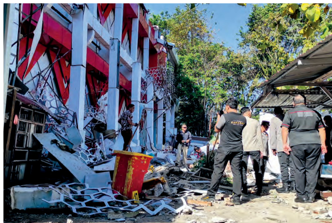
Police officers look at a building of the North Sumatra's National Sports Committee of Indonesia (KONI) damaged following a severe 7.4-magnitude offshore quake in Manado, North Sulawesi
