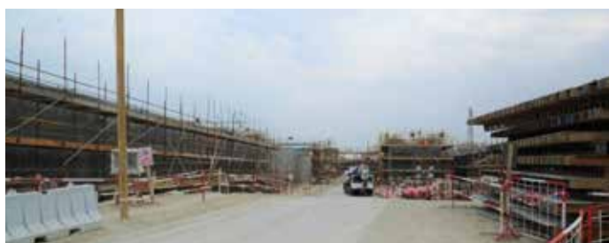
Construction work in progress
