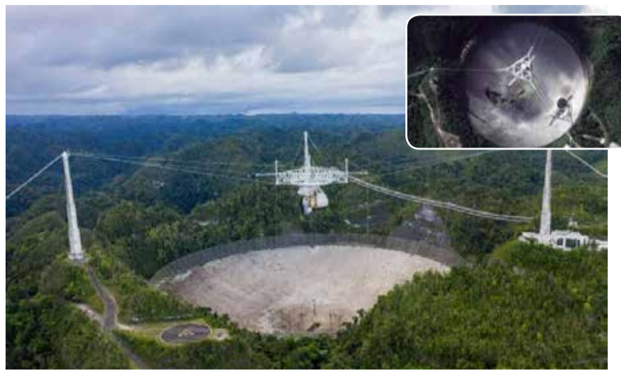
The Arecibo Observatory in Arecibo, Puerto Rico, before its collapse. Inset, a hole in the dish panels of the Arecibo Observatory in Arecibo, Puerto Rico, last month after a cable snapped and gashed the reflector disc
