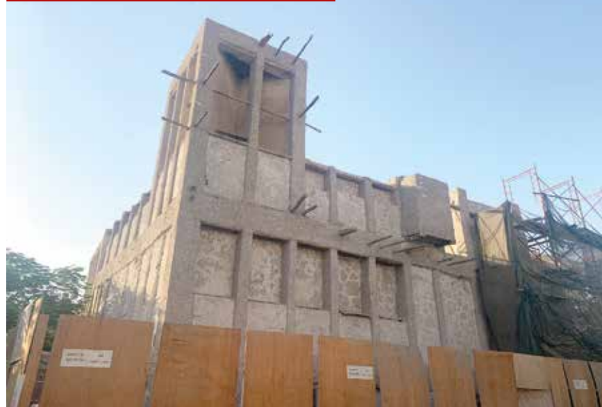
One of 5 of the last surviving traditional wind towers, a traditional form of air-conditioning, in Bahrain at Al Alawi House. Pictures tweeted by @AhamadNooh. The wind tower functions as a Solar or thermal chimney that uses convection of air heated by passive solar energy. It creates a pressure gradient which allows less dense hot air to travel upwards and escape out the top.
