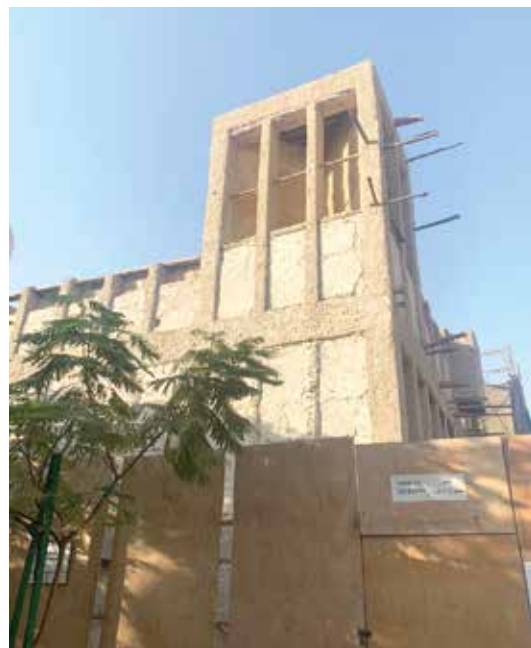
One of 5 of the last surviving traditional wind towers, a traditional form of air-conditioning, in Bahrain at Al Alawi House. Pictures tweeted by @AhamadNooh. The wind tower functions as a Solar or thermal chimney that uses convection of air heated by passive solar energy. It creates a pressure gradient which allows less dense hot air to travel upwards and escape out the top.
