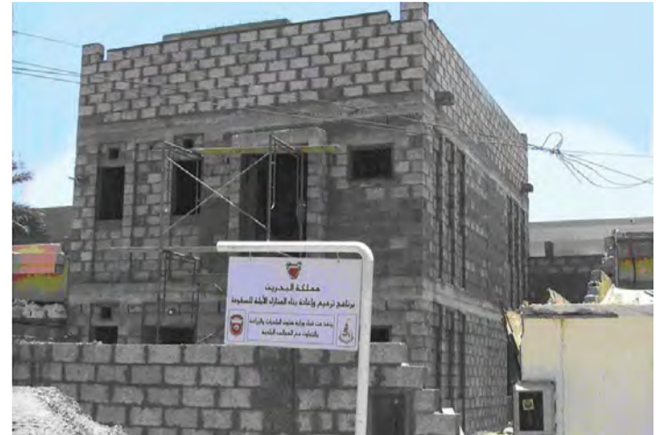
A residential home undergoes reconstruction under Bahrain's approved housing support plan
