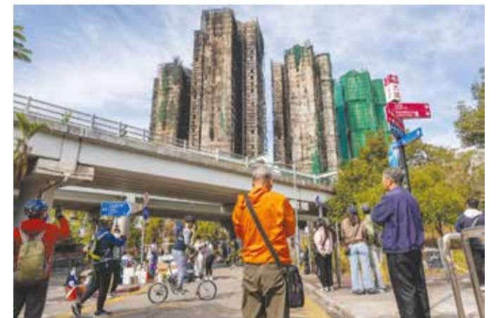
People look at the aftermath of a major fire that swept through several apartment blocks at the Wang Fuk Court residential estate in Hong Kong's Tai Po district
